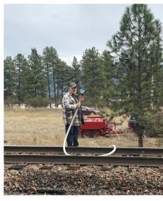
train had ran over this section of track earlier in the day grinding the rails, which is what ignited the railway ties. This, apparently, is not an uncommon occurrence!
