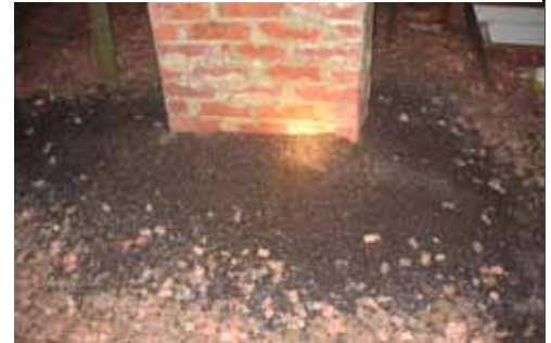
Accumulation of guano (bat droppings) around a chimney in an attic can be cleaned annually to reduce smell.
